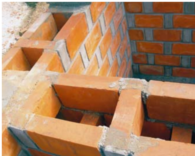
Better building methods can improve the energy efficiency of buildings: this rat trap bond masonry saves bricks and insulates better
