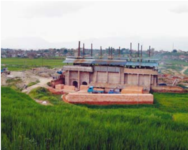
The Vertical Shaft Brick Kiln (VSBK) is the most efficient brick kiln; it saves up to 40% coal compared to conventional kilns
